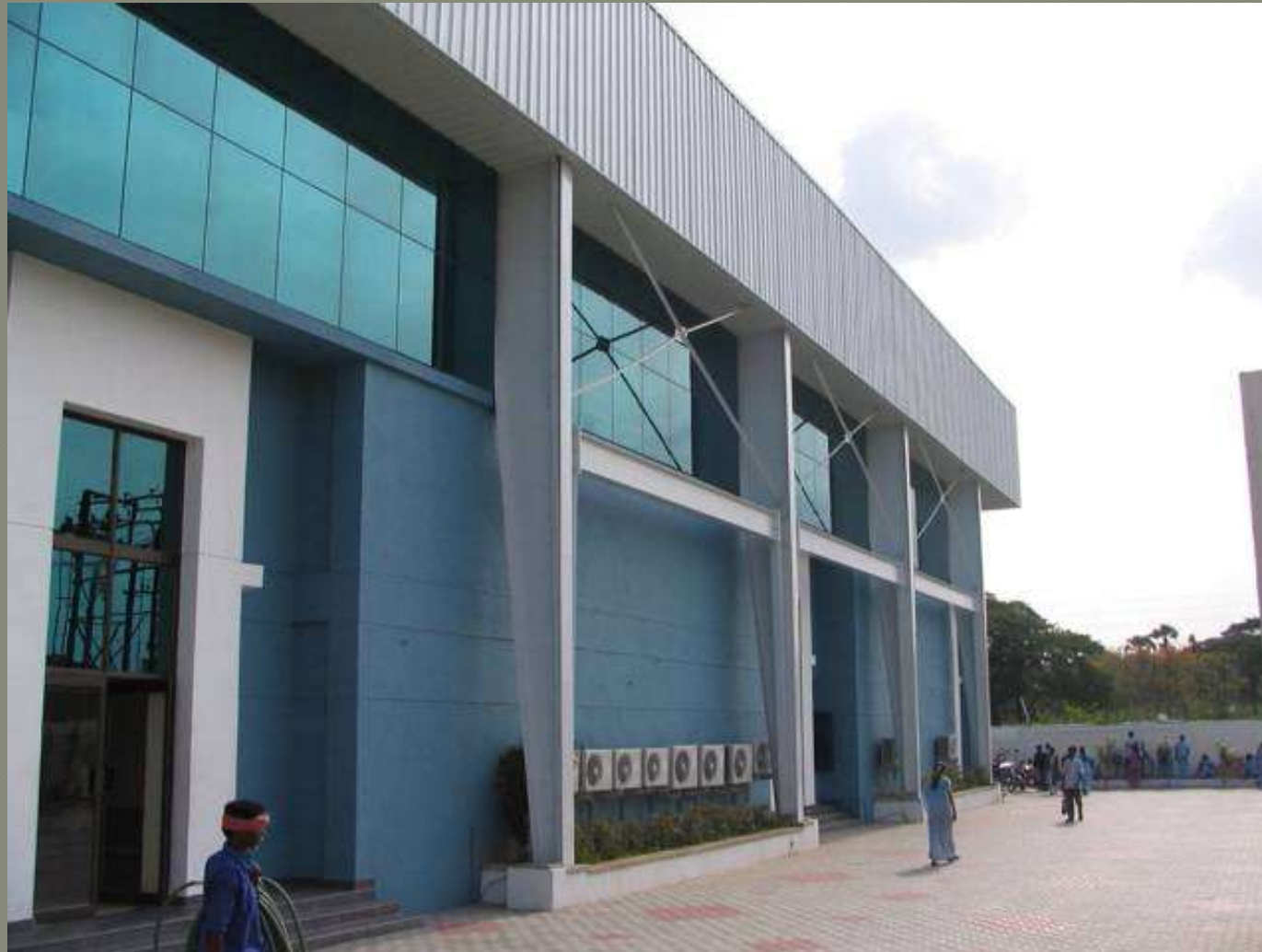
Unusual Full height brick wall with exterior visible main frame columns
